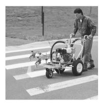
LineLazers are three times faster than air spray striping and twice as fast when compared to other airless stripers!
