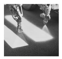
Unlike air spray stripers, the LineLazer delivers high quality lines with squared beginnings and ends, razor sharp line edges and perfectly uniform paint distribution across the line.
